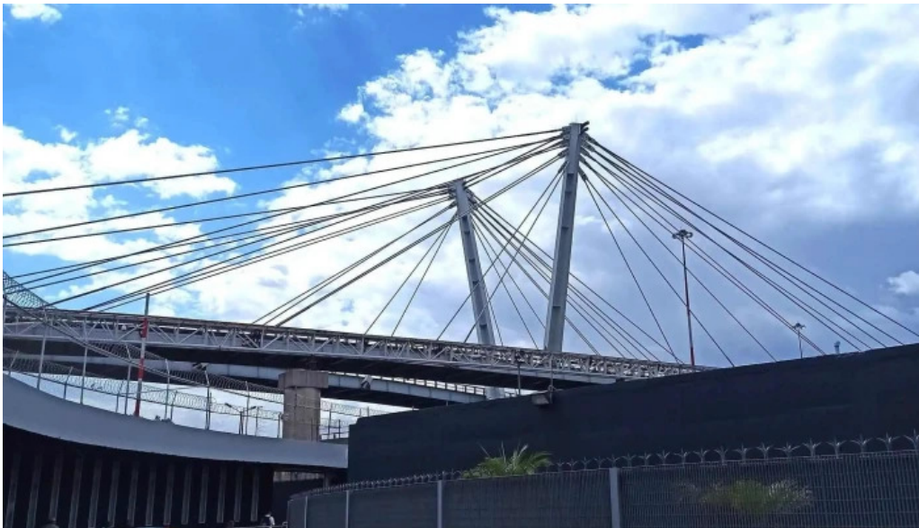
Terminal aerea comentarios
