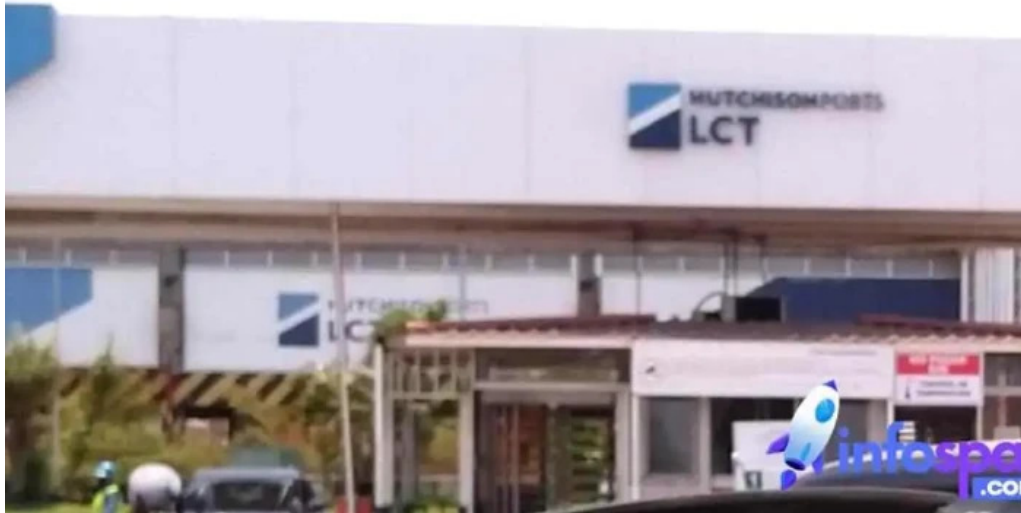
Hutchison ports lct exterior
