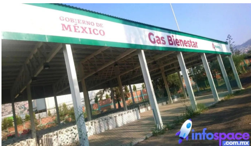
Tad satellite norte san juan ixhuatepec pemex logistica exterior
