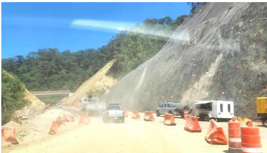
Tunel san sebastian coatlan km 51726 long 168 m horario
